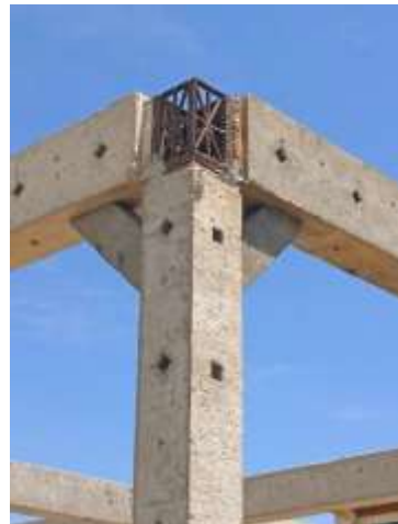
Connection between 1 column and 2 beams.
