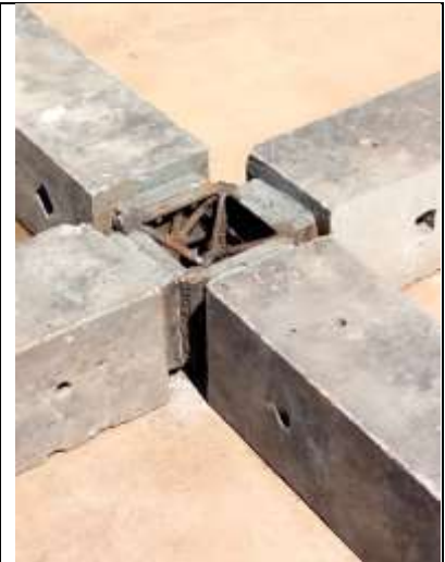
Connection between 4 adjacent beams.
