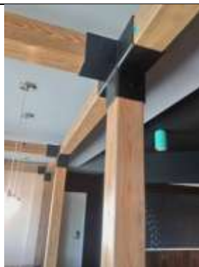
Similarity: steel connection in wood construction.
