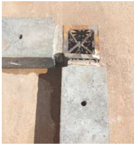
Connection between 2 adjacent beams
